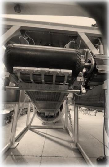
Weighing and inclined belts
